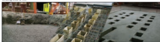
Concrete pad for specialized equipment at plant.
