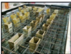
Formwork that was constructed for a concrete base for specialized equipment.
